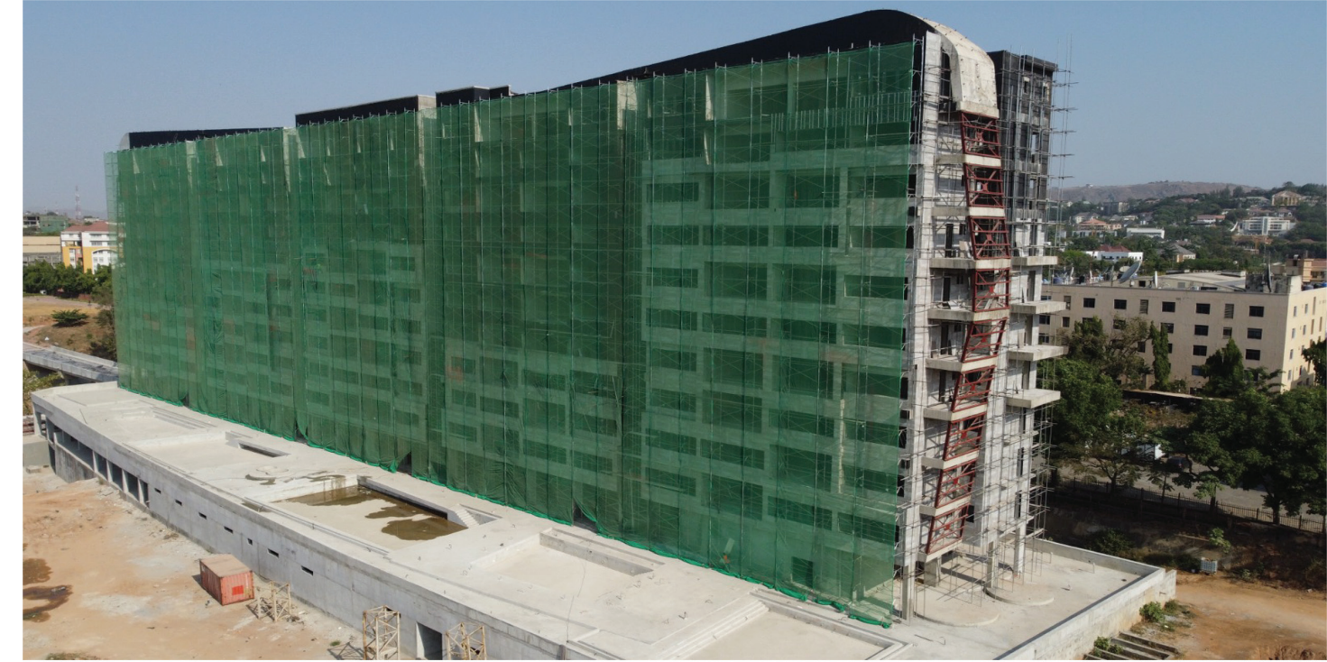
Image: Jibike's Luxury Apartments Project Progress January 2025
