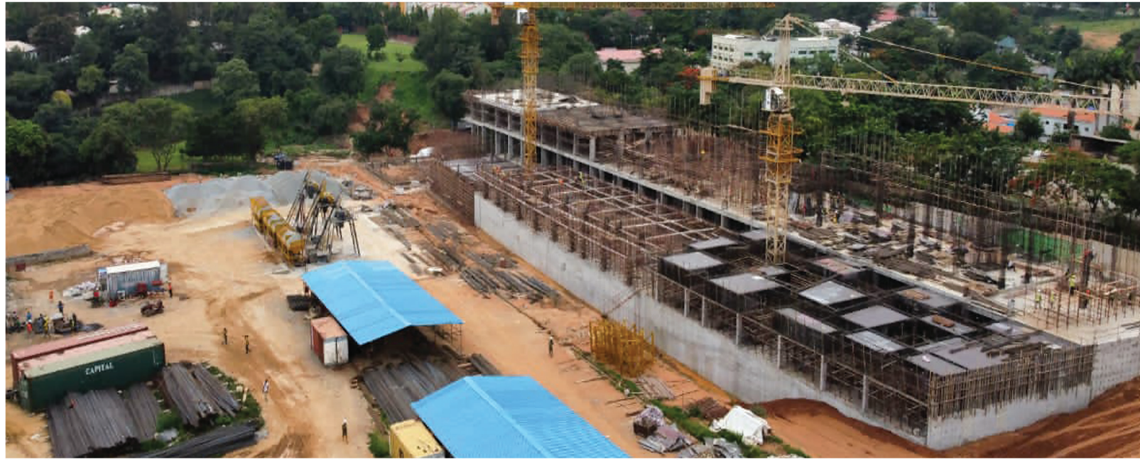
Image: Jibike's Luxury Apartments Under construction July 2022
