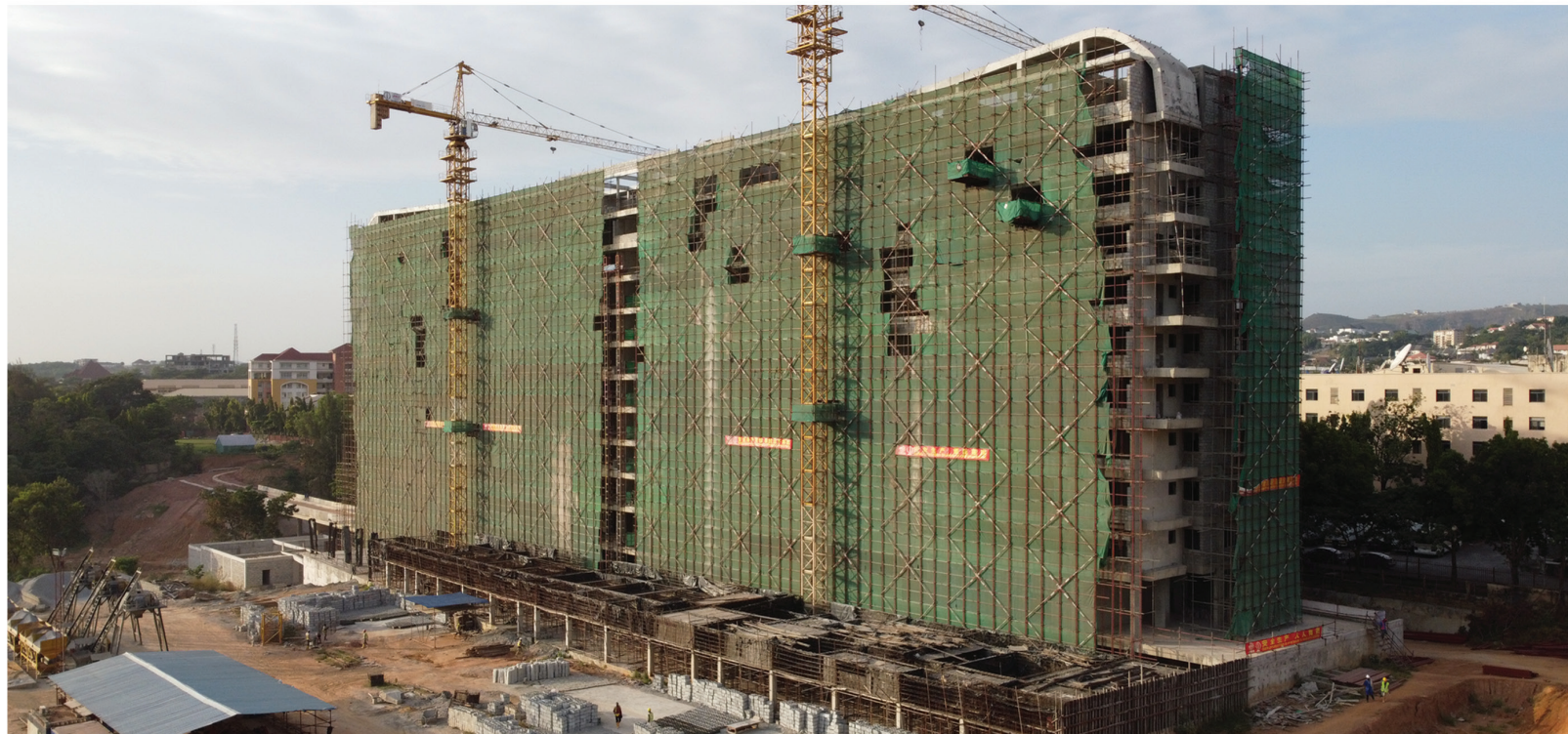
Image: Jibike's Luxury Apartments Project Progress November 2023
